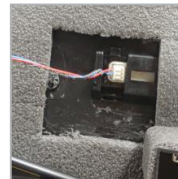
② Make clean the surface
