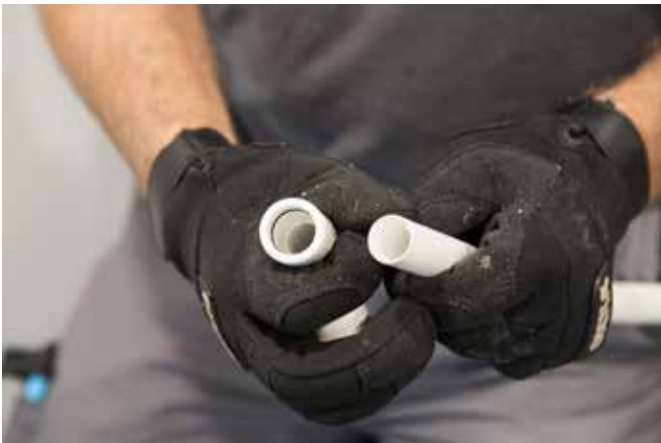
• STEP 3: PRE-MOUNTED O-RING AND PRE-LUBRICATED
