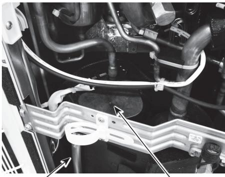
Compressor lead wire Terminal cover
