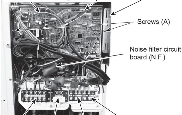
Terminal block (TB1)    Terminal block (TB1B)    Terminal block (TB3)    Terminal block (TB7)
